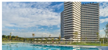
BeCasa Alcobendas, Sant Cugat, Baraka (BTR)
