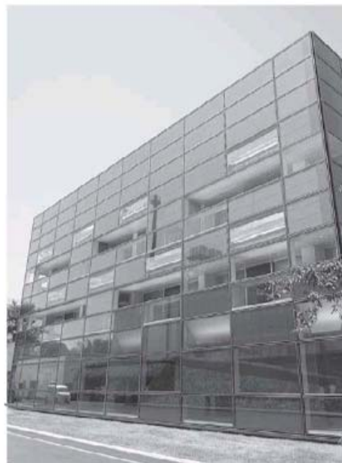
This Taisei office in Yokohama uses solar panels on the sides and roof.
